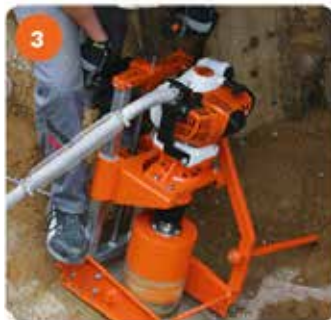
90° Drill in sewage pipe. Pipe base clamped between concrete pipe and trench and secured by ground spikes.
