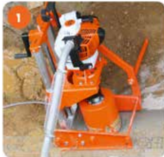
90° Drill in sewage pipe. Pipe base clamped between concrete pipe and trench and secured by ground spikes.
