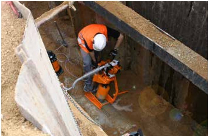
90° Drill in sewage pipe. Fixing by ground spikes
